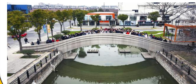
3D-Printed Concrete Pedestrian Bridge Completed in China (2018)
