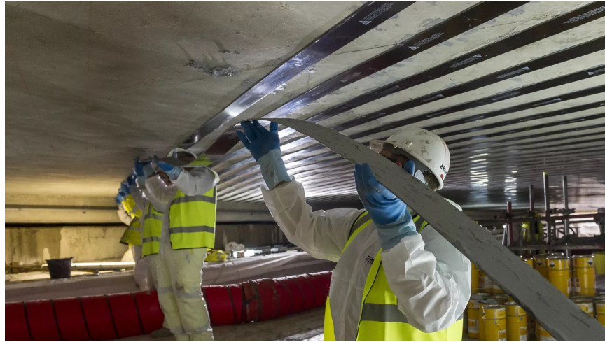
Figure 1.2: Installation of Sika's CFRP plates for building support [33]
