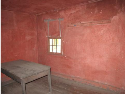
4.42 K203-II-3. West wall, on grayish ghost behind position for former curtain support for comparison Visible Light 200X
