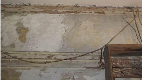
4.36 K101-II-16. Board just above pegrail used to support gas pipe and later support water pipe, on south wall just above door Visible Light 40X
