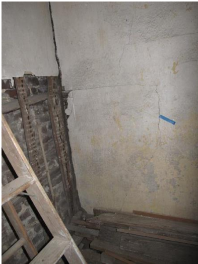
4.40 K104-II-3. South wall, southeast corner, at crack about 4' up Visible Light 100X
