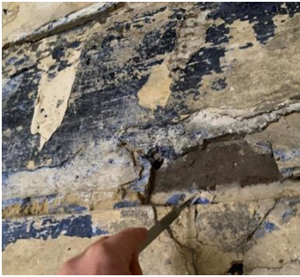
4.58 K-3. Kitchen, north wall on shelf ghost. Detached paint flake from substrate Visible Light 100X
