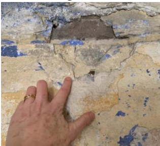
4.57 K-2. Kitchen, north wall, second generation of plaster near K-1. Later generation of plaster, starting at layer 23 Visible Light 100X
