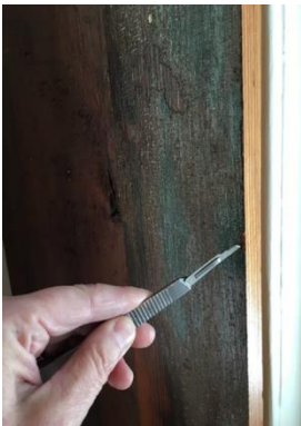
4.68 5. Reused board on shutter, may have been from door, on paint remnants Visible Light 100X
