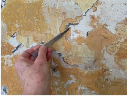
4.62 L-1. North wall, yellow limewash under blue, east side Visible Light 100X
