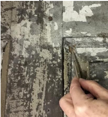
4.53 2-5. 2 nd fl. Door to east room, passage side, upper right corner of middle right panel Visible Light 200X
