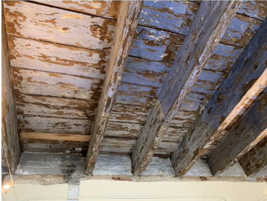
Figure 2.5 Image by Dr. Susan Buck. Ceiling and west wall of first floor Carriage House with partition ghosts.
