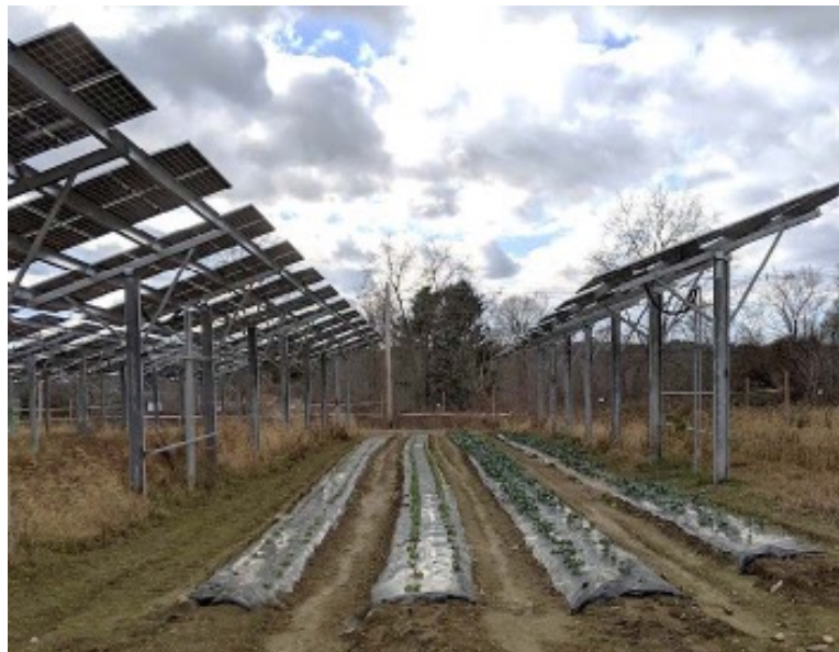
Figure 1. Lettuce production under agrivoltaic installation. Photo credit: Sam Glaze-Corcoran
